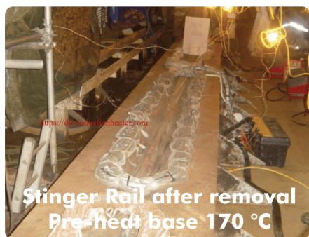
Structural: rail base preheated to 170 °C.
