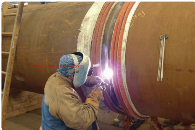
Large-diameter line pipe with induction cable during welding.
