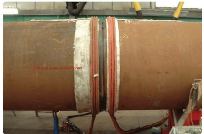
Two joints prepared with insulation and induction cable.
